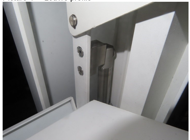
Picture 6 Louvre mechanism
