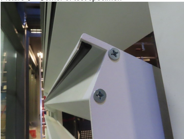
Picture 5 Louvre sealing gasket
