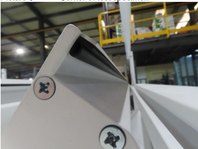
Picture 5 Louvre sealing gasket
