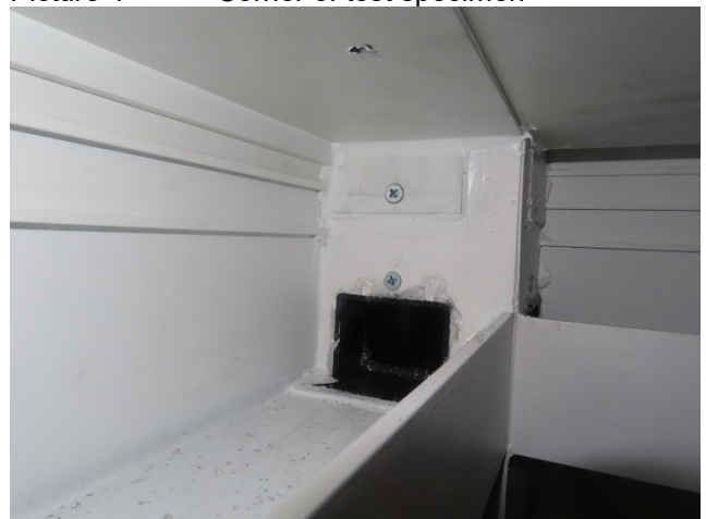
Picture 6 Drainage system
