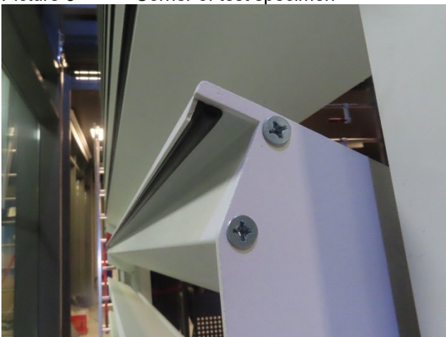
Picture 5 Louvre sealing gasket
