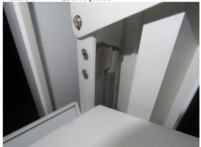
Picture 6 Louvre mechanism
